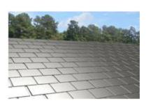
**Shingles, Aluminum:** A roof cover made of aluminum shingle tiles with interlocking side laps or side joints. Assumes custom roof material colors and patterns.
