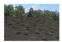
Shingles, Asphalt/Fiberglass, Irregular Pattern: A roof cover made up of architectural asphalt/fiberglass shingles with multi-layered construction where random tabs or pads are applied to a base shingle to achieve added dimension and custom patterns. These shingles are sometimes referred to as laminated or three-dimensional shingles. Assumes custom roof material colors and patterns typical of high value homes.
