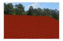
**Shingles, Slate Red:** A roof cover of shingles made from red slate, a fine-grained metamorphic rock produced by the compression of various sediments cut into thin tiles or slabs. Assumes custom roof patterns typical of high value homes.
