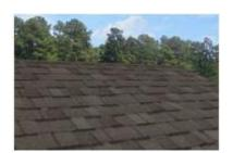
**Hail Proof:** A roof cover made of high impact laminated asphalt shingles. The shingles are composed of a heavyweight, non-woven fiberglass mat which is thoroughly impregnated and coated with modified asphalt for superior strength. Assumes custom roof material colors and patterns typical of high value homes.
