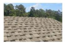
Shingles, Architectural: Designer asphalt/fiberglass shingles featuring multi-layered construction, where random tabs or pads are applied to a base shingle to achieve added dimension and replicate the look of wood shakes. These shingles are sometimes referred to as laminated or three-dimensional shingles. Assumes custom roof material colors and patterns typical of high value homes.
