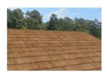
**Shakes, Wood:** Shakes split from a bolt of wood, generally in random dimensions. Wood shakes are normally installed over a pitched roof on spaced sheathing covered with a vapor barrier. Assumes custom roof material colors and patterns typical of high value homes.
