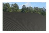
**Tin (Terne):** A thin gauge sheet of tin (terne) that is typically fastened with a standing seam system. Tin alloys have a long life span and are a premium cost product. Tin roofs are not to be confused with the steel roofs commonly found on pre-engineered structures. Assumes custom roof material colors and patterns typical of high value homes.
