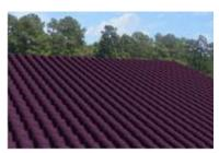
**Tile, Clay, Custom Colors:** A roof cover made of tapered or straight clay roofing tiles that are either barrel shaped or S-shaped with interlocking side laps/side joints and have a unique coloring. Assumes custom roof patterns typical of high value homes.
