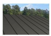
**Tin, Lead Coated Standing Seam:** A roof cover that is made of tin, a white malleable metal that is highly resistant to corrosion which contains a lead coating, connected with interlocking seams that are raised above the drainage plane and form a seal. Assumes custom roof material colors and patterns typical of high value homes.
