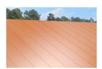
**Copper, Flat Seam:** A roof cover made of sheets of copper connected with interlocking flat seams. Assumes custom roof material colors and patterns typical of high-value homes.
