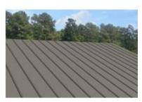
**Terne, Batten Seam:** A roof cover made up of sheets of steel or iron coated with a terne alloy (80% lead and 20% tin), making it highly resistant to corrosion. The pieces are connected with standing seams or interlocking seams raised above the drainage plane forming a seal. With the addition of snap-on batten seam covers, the roof has a pronounced standing-seam appearance. Assumes custom roof material colors and patterns typical of high value homes.
