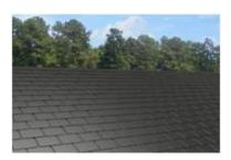
**Shingles, Steel:** A roof cover made up of steel roofing shingles. Assumes custom roof material colors and patterns typical of high value homes.
