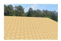
**Shakes, Victorian Scalloped:** Wood shakes split from a bolt of wood and cut into the scalloped shape typical in Victorian homes. Assumes custom roof material colors and patterns typical of high value homes.
