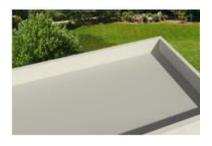
**Foam:** A sprayed polyurethane foam (SPUF) roof sprayed on the substrate, forming a single continuous structure that is seamless and very stable. Assumes custom roof material colors and patterns typical of high value homes.
