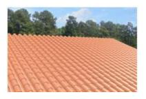
**Tile, Clay, Glazed:** A roof cover made of tapered or straight glazed clay roofing tiles that are either barrel shaped or S-shaped with interlocking side laps/side joints and have a standard and/or custom coloring. Roof tiles are traditionally fired in kilns to dry. Assumes custom roof patterns. Also known as Oriental or Japanese tile roofing.
