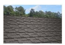
**Shingles, Steel, Aggregate Finish:** A roof cover made up of steel roofing shingles that are surfaced with mineral granules. Assumes custom roof material colors and patterns typical of high value homes.
