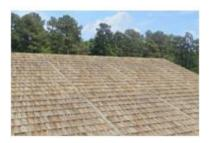
**Shingles, New England Pine:** Overlapping tapered pieces of New England pine, generally in random dimensions. New England pine shingles are installed over a pitched roof on spaced sheathing covered with a vapor barrier. Assumes custom roof material colors and patterns typical of high value homes.
