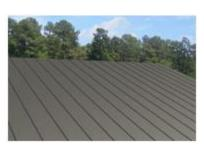
**Aluminum, Standing Seam:** A roof cover made of roll-formed aluminum panels with raised seams above the drainage plane forming a seal. Assumes custom roof material colors and patterns.
