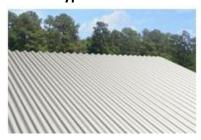
**Aluminum, Corrugated:** A roof cover made of corrugated aluminum sheets applied over a pitched roof. Assumes custom roof material colors and patterns.
