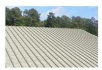
**Tile, Concrete:** A thin piece of concrete made from Portland cement, fine aggregate, and pigments. Assumes custom roof material colors and patterns typical of high value homes.
