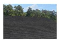
**Slate, Reinforced Fiber Composite:** A roof cover made of non-asbestos fiber reinforced cement slates with a uniform thickness of 1/4". The slates are produced under compression with an integrated slate/green color finish and have an authentic slate texture with beveled edges. Assumes custom roof patterns typical of high value homes.
