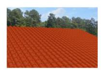
**Tile, Clay:** A roof made from different types of clay and fired in kilns to dry. Clay tiles can be divided into two categories: flat or roll.
