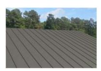
**Tin, Lead-Coated, Batten Seam:** A roof cover that is made of tin, a white malleable metal that is highly resistant to corrosion which contains a lead coating and includes snap-on batten seam covers. Assumes custom roof material colors and patterns typical of high value homes.
