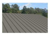
**Steel:** A roof cover of corrugated steel sheets applied over a pitched roof.
