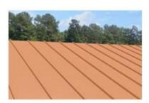
**Copper, Batten Seam:** A roof cover made up of sheets of copper connected with standing seams or interlocking seams raised above the drainage plane forming a seal. With the addition of snap-on batten seam covers, the roof has a pronounced standing-seam appearance. Assumes custom roof material colors and patterns typical of high-value homes.
