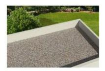
**Built-Up/Tar and Gravel:** Three to five layers of roofing felt laminated with coal tar, pitch or asphalt and topped with a layer of gravel or other aggregate material. Typically found on flat or low-pitched roofs. Assumes custom roof material colors and patterns typical of high value homes.
