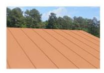
**Copper, Standing Seam:** A roof cover made of sheets of copper connected with interlocking seams that are raised above the drainage plane, forming a seal. Assumes custom roof material colors and patterns typical of high value homes.
