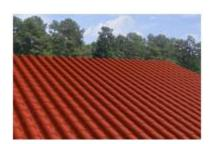
**Tile, Mission:** Barrel shaped mission clay tile roofing applied over asphalt felt. Assumes custom roof material colors and patterns typical of high value homes.
