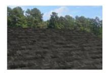
**Slate:** A dense, fine grained, metamorphic rock produced by the compression of various sediments, cut into thin tiles or slabs. Slate comes in many sizes, thicknesses and finishes. Assumes custom roof patterns typical of high value homes.
