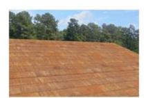
Shingles, Wood, Fire Resistant: A roof cover made of wood shakes/shingles that are treated with a fire-retarding chemical and are pressure-treated to impregnate the retardant into the inner cells of the wood, resulting in a fire-resistant product. Assumes custom roof material colors and patterns typical of high value homes.
