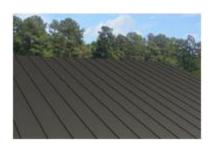
**Terne, Standing Seam:** A roof cover made up of sheets of copper connected with standing seams or interlocking seams raised above the drainage plane forming a seal. With the addition of snap-on batten seam covers, the roof has a pronounced standing-seam appearance. Assumes custom roof material colors and patterns typical of high-value homes.
