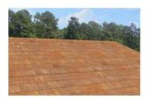
**Shingles, Wood:** Overlapping, tapered pieces of wood, generally in random dimensions. Wood pine shingles are installed over a pitched roof on spaced sheathing covered with a vapor barrier. Assumes custom roof material colors and patterns typical of high value homes.
