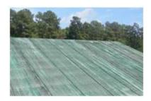
**Copper:** Sheets of 16 oz. copper connected with interlocking seams used to cover pitched roofs. The seams are either flat or raised. Assumes custom roof material colors and patterns typical of high value homes.
