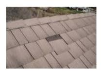
**Masonite:** A roof cover made up of fiberboard products consisting of pressure bonded fibers designed to resemble natural cedar roofing or wood shake or shingle roofing.
