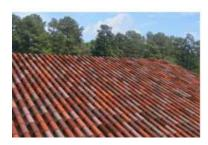
**Tile, Spanish:** Clay tiles that are S-shaped with interlocking side laps or side joints. Assumes custom roof material colors and patterns typical of high value homes.
