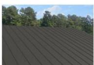
**Steel, Standing Seam:** A roof cover made of roll-formed steel panels with raised seams above the drainage plane forming a seal. Assumes custom roof material colors and patterns.
