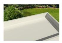
**Vinyl:** A single ply reinforced vinyl (polyvinyl chloride) fabric membrane used as a roof covering material. Seams are heat welded to create a continuously sealed vinyl membrane that covers the roof. The roof membrane contains a fabric or fiber reinforcement material, vinyl resins, ultraviolet light and heat stabilizers, bactericides, coloring agents, and polymers. Typically found on flat or low pitched roofs.
